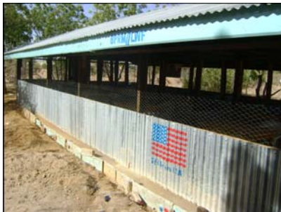
Shed for Social assessment at Dagahaley Camp
